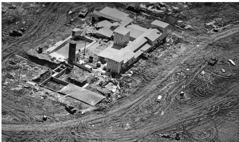
Photo 2. A tank on 19 April 1993 is seen entering the front of the residence, apparently aiming for the concrete vault at the base of the central tower. The gymnasium in the back of the building has been demolished by another tank. Government exhibit in the 2000 civil trial.
