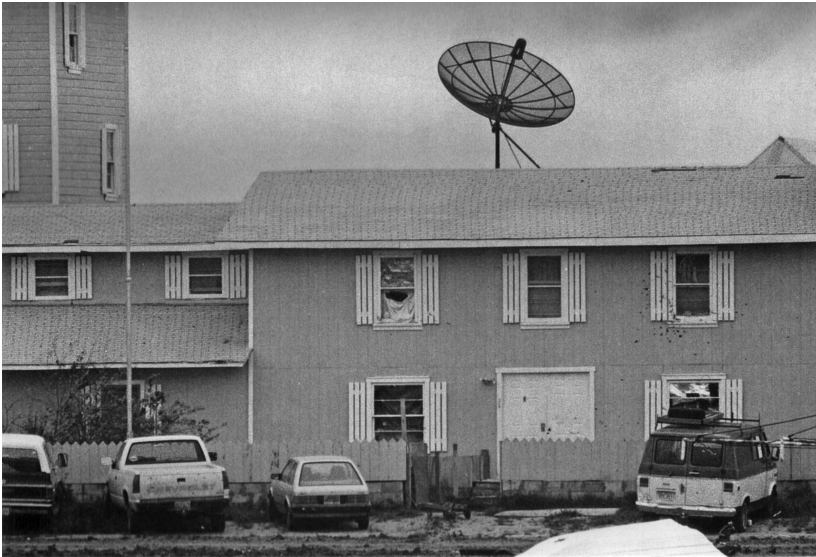
Photo 1. The front of the Mount Carmel residence after the shootout with ATF agents on 28 February 1993. Bullet holes are visible in the walls, around the windows, and especially around the right-hand side of the double front door. Government exhibit in the 2000 civil trial.
