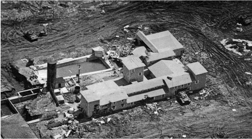
Photo 3. The tank in the front of the building has relocated east to enter the building at the double front doors. A tank will begin to enter the building from the back. Attorney David Hardy alleges that the tanks were aiming for David Koresh and Steve Schneider on the second floor. Government exhibit in the 2000 civil trial.
