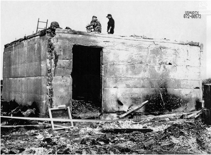
Photo 8. The concrete vault after the fire. The small flags mark where bodies or body parts were located. Government exhibit in the 2000 civil trial.
