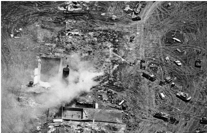
Photo 7. An aerial shot shows that a fire truck was not permitted to start spraying water until after the residence had burned down completely. Government exhibit in the 2000 civil trial.
