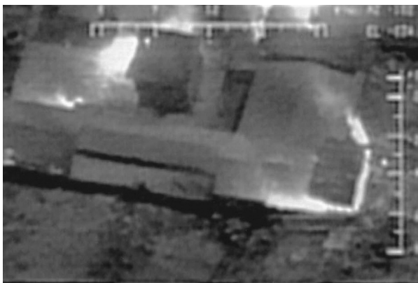
Photo 5. FLIR imagery shows that at 12:11 A.M. the fire on the front southeast corner has spread to the chapel, and that there are fires in the back in the gymnasium, and in the kitchen area to the west side of the tower. Government exhibit in the 2000 civil trial.
