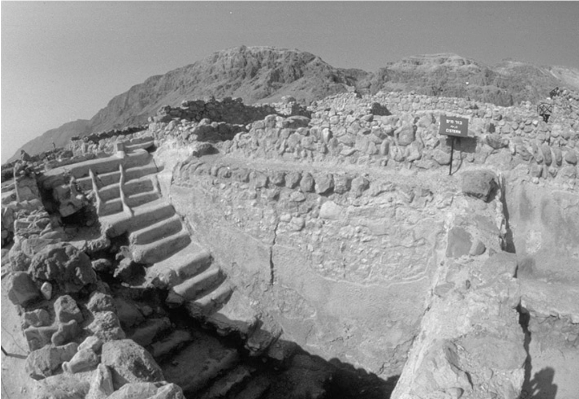
Ritual Bath (damaged by an earthquake) at Kh. Qumran
